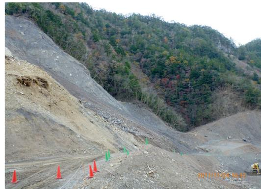
Photo 4 A spill way under construction at the Nagatono landslide dam site. The photo was taken in Nov. 24, 2011.
