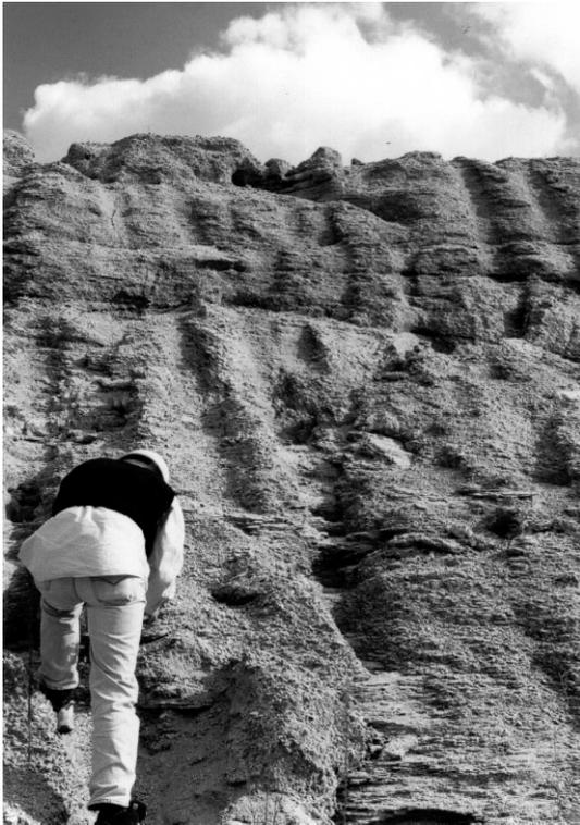
Fig. 7. Typical occurrence of micro-sheeting in a cut slope at Seifu-Shinto. The micro-joints strike parallel to the cut slope and dip downslope.
