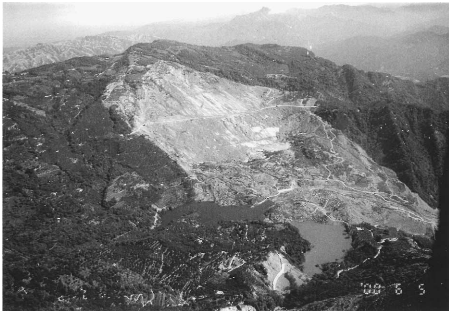
Fig. 1. Overview of the Chiu-fen-erh-shan landslide, looking to the southeast.
